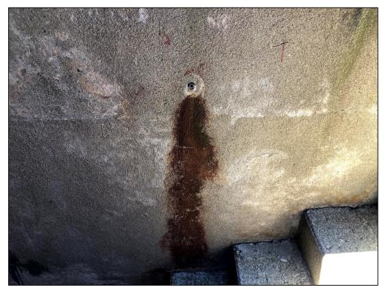
Photo 17: Apparent pipe with evident rust staining in exterior stairwell.
