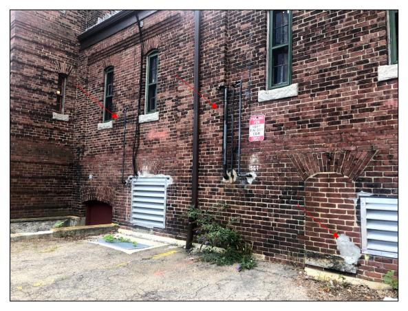
Photo 16: Series of 4 vent pipes along eastern building exterior, adjacent to closed AST fill pipe.
