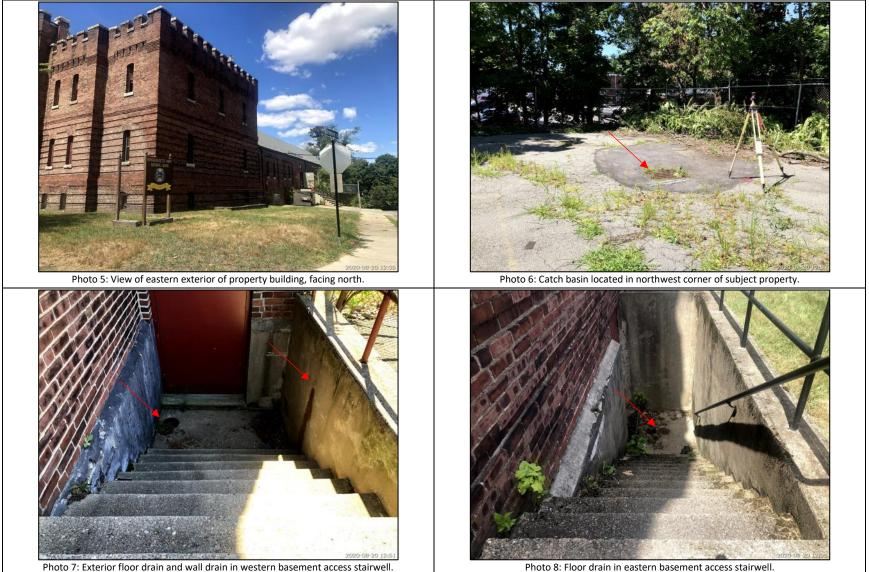
Photo 8: Floor drain in eastern basement access stairwell.
