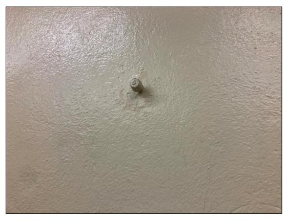
Photo 7: Capped piping. Eastern interior Wall of kitchen – basement.
