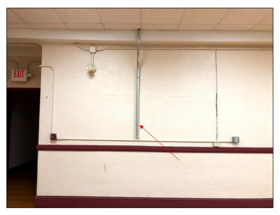
Photo 3: Possible floating electrical conduit line
