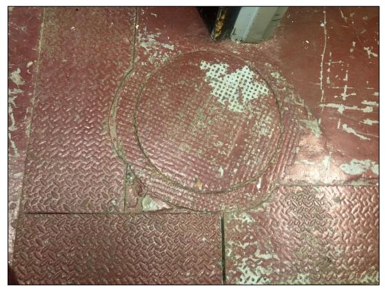
Photo 15: Trench plating and drainage system cap (manhole cover, one of several in basement)
