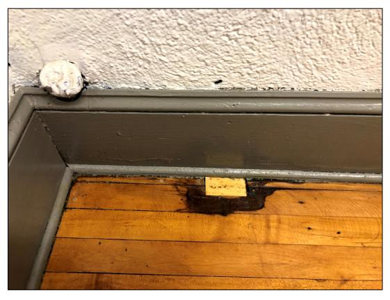
Photo 5: Disconnected, plugged piping in admin upper level admin area.
